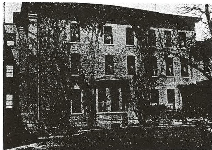
The Old Dormitory Built in 1875
